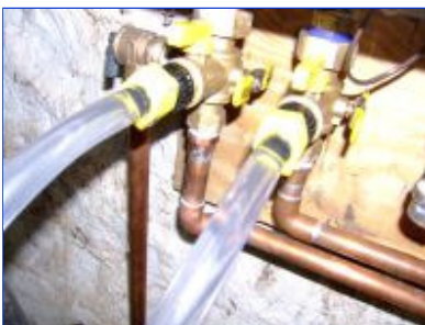
Valve drain caps removed, vinyl tubes with garden hose fittings screwed onto drain ports, water inlet/outlet valves closed, drain valves opened. Tube from transfer pump connected to cold water side, discharge from hot water side.
